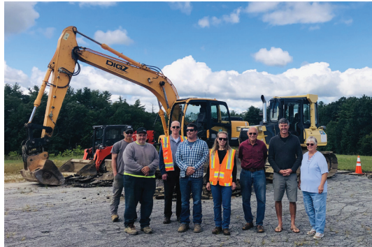
Ground Breaking, Friday, September 3, 2021
